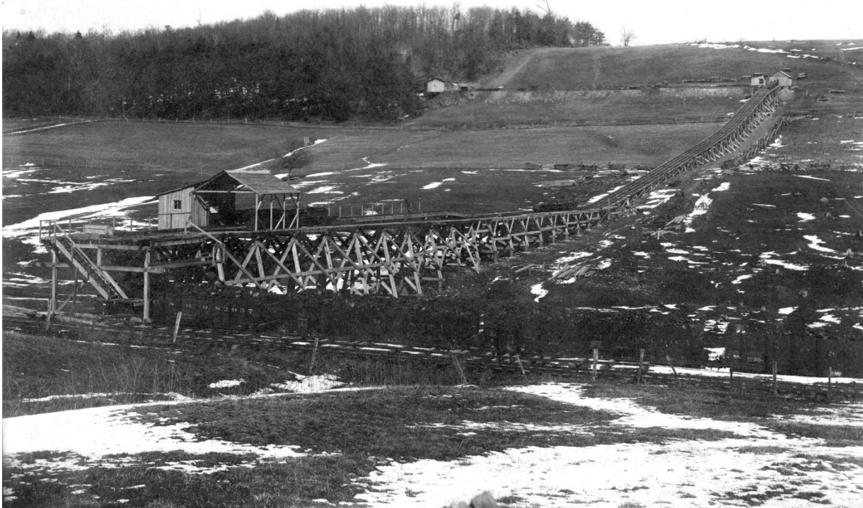
Glenwood Coal Company, Rickertsdale Tipple in Glen Campbell, Indiana County, Pennsylvania, circa 1900
